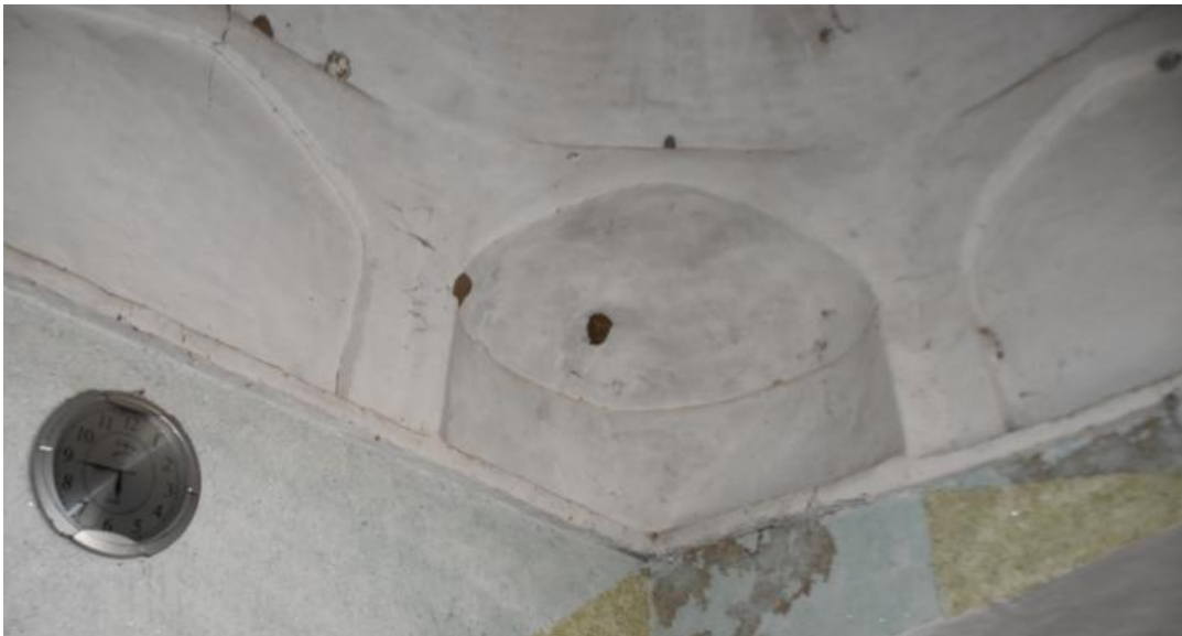
Figure 35: Interior view of Giri Mosque
