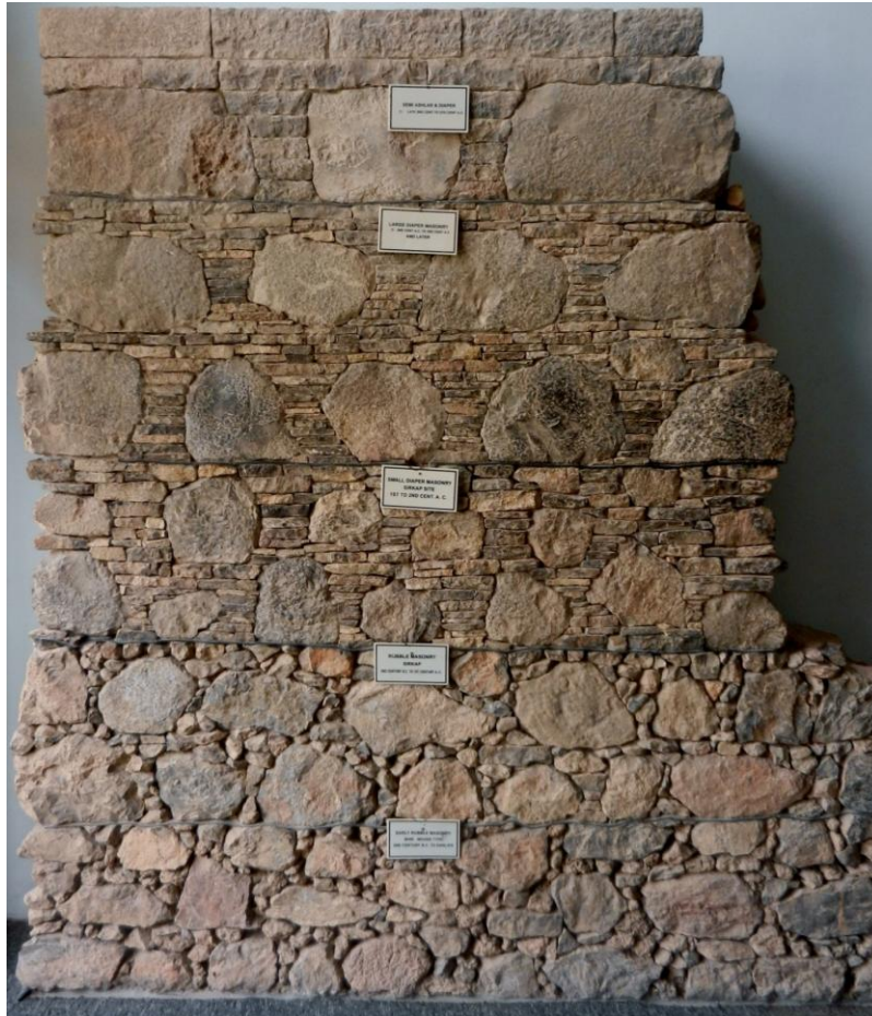
Figure 49: Levels of Construction in the cities and monuments of Taxila from oldest (at bottom) to latest (at top)
