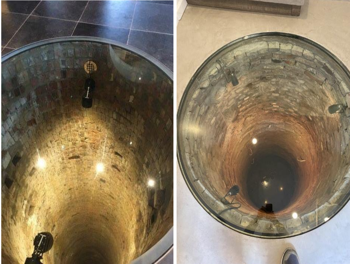
Figure 22: References for preserving and sealing these wells while retaining their historical significance
