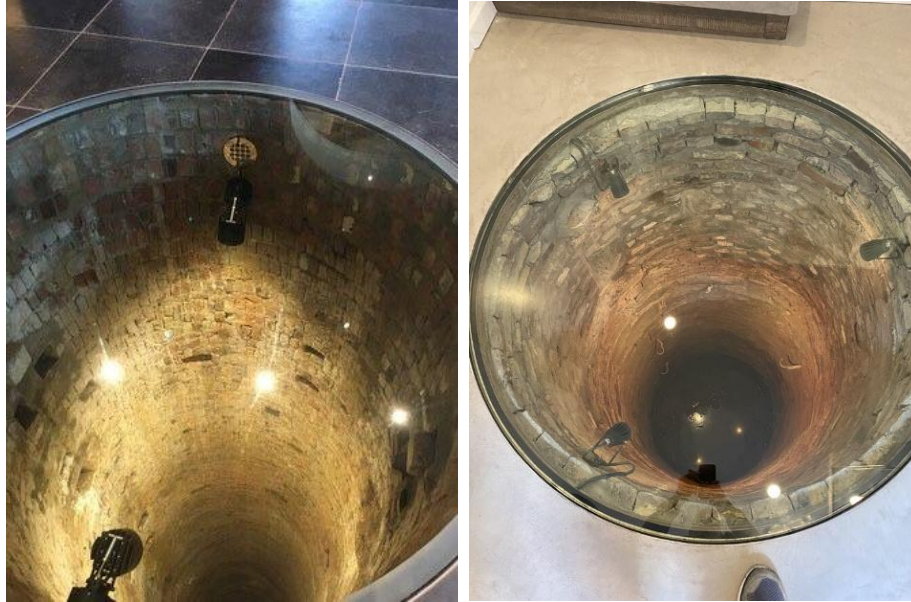
Figure 10: References for preserving and sealing these wells while retaining their historical significance
