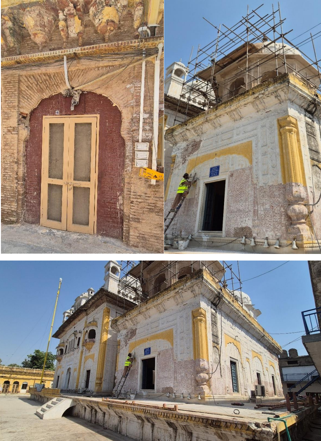
Figure 31: Ongoing conservation works on site expected to be completed in 2026
