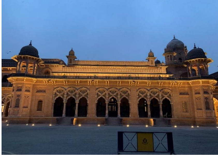
Figure 15: Side elevation, Aitchison's old building
