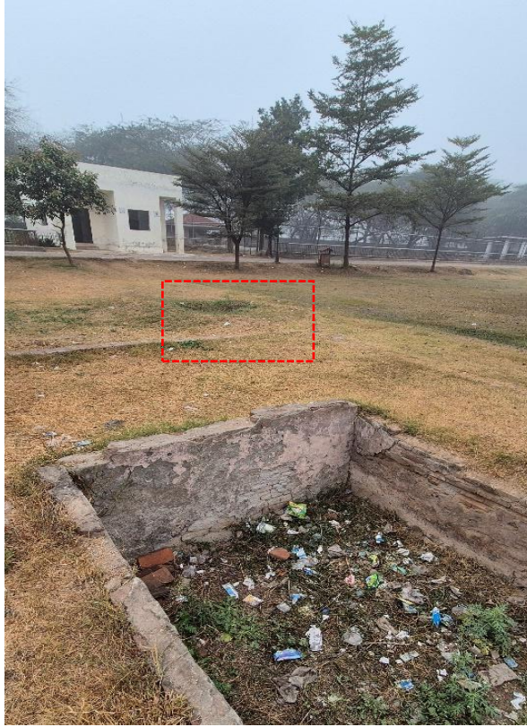
Figure 12: Water channel in the lawn of Hiran Minar, blocked by solid waste
