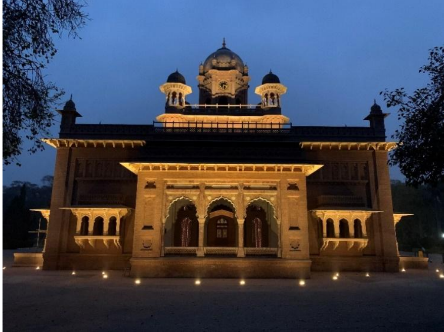
Figure 17: Rear elevation, Aitchison's old building
