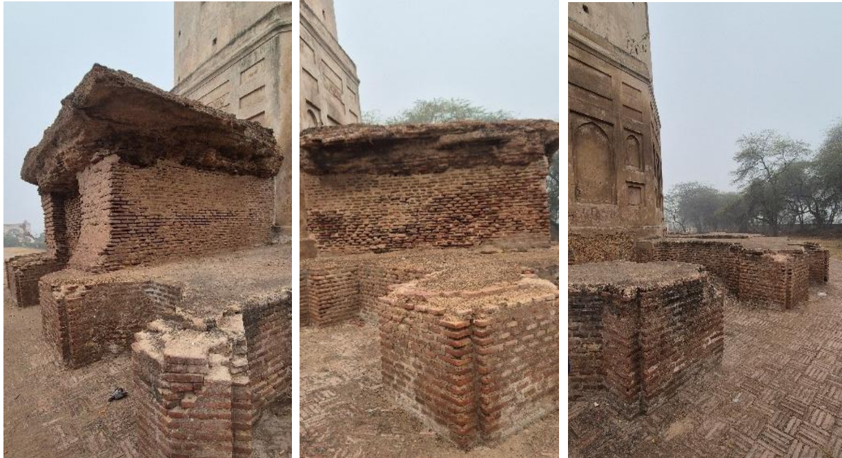
Figure 21: Existing condition of Hiran Minar
