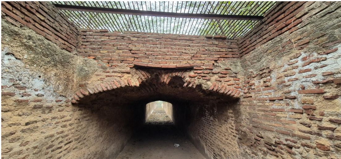
Figure 12: Water channel in the lawn of Hiran Minar, blocked by solid waste
