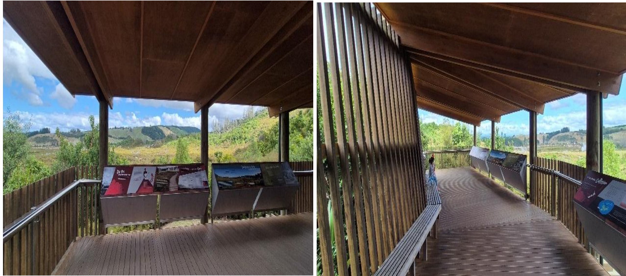
Figure 7: Reference images for introducing a deck on site
