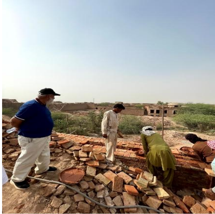
Figure 16: Urban Unit team inspecting the ongoing restoration work of boundary wall
