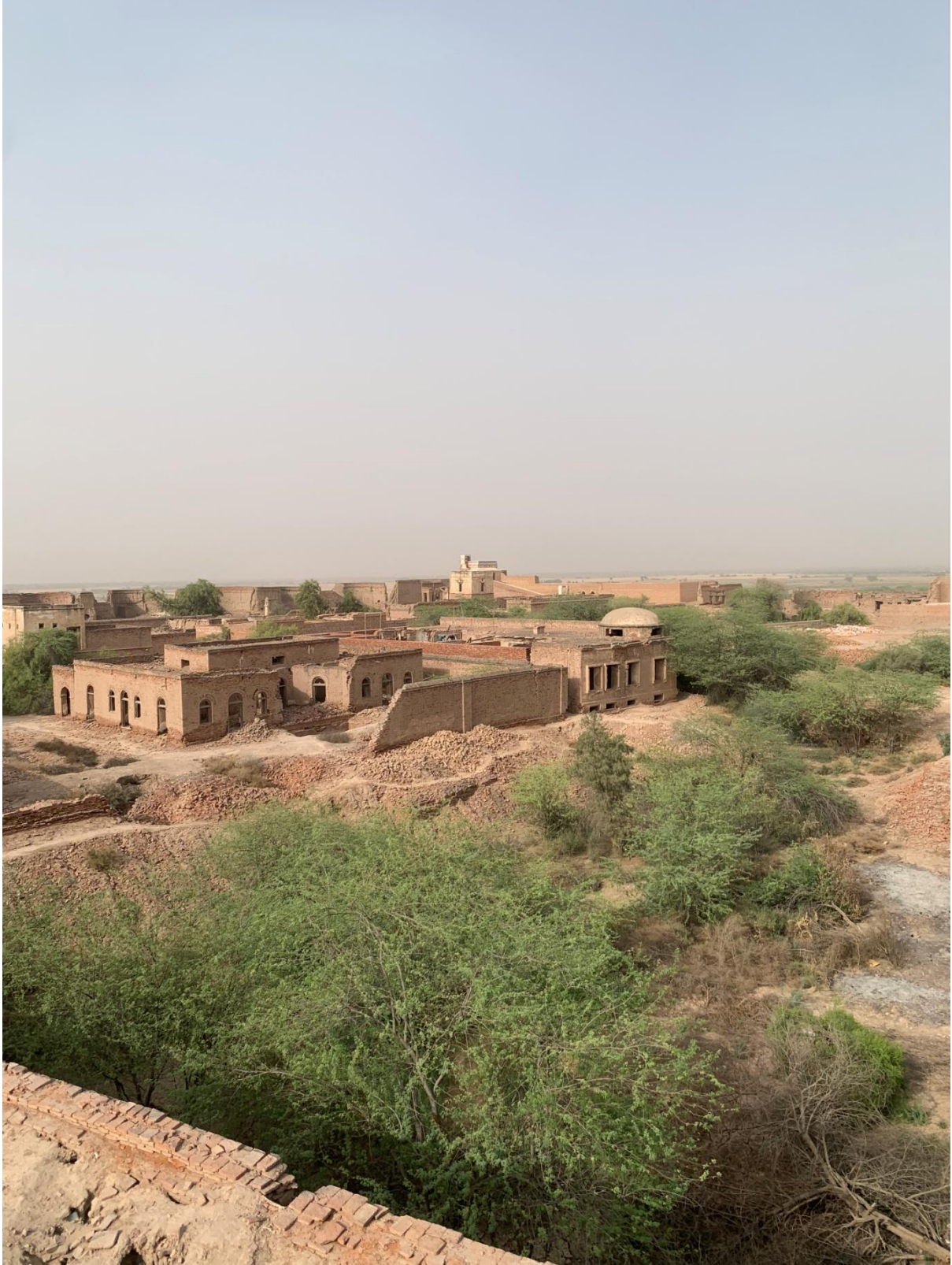
View of Pond from bastions in background fallen wall and sinking buildings of Haram are visible.
