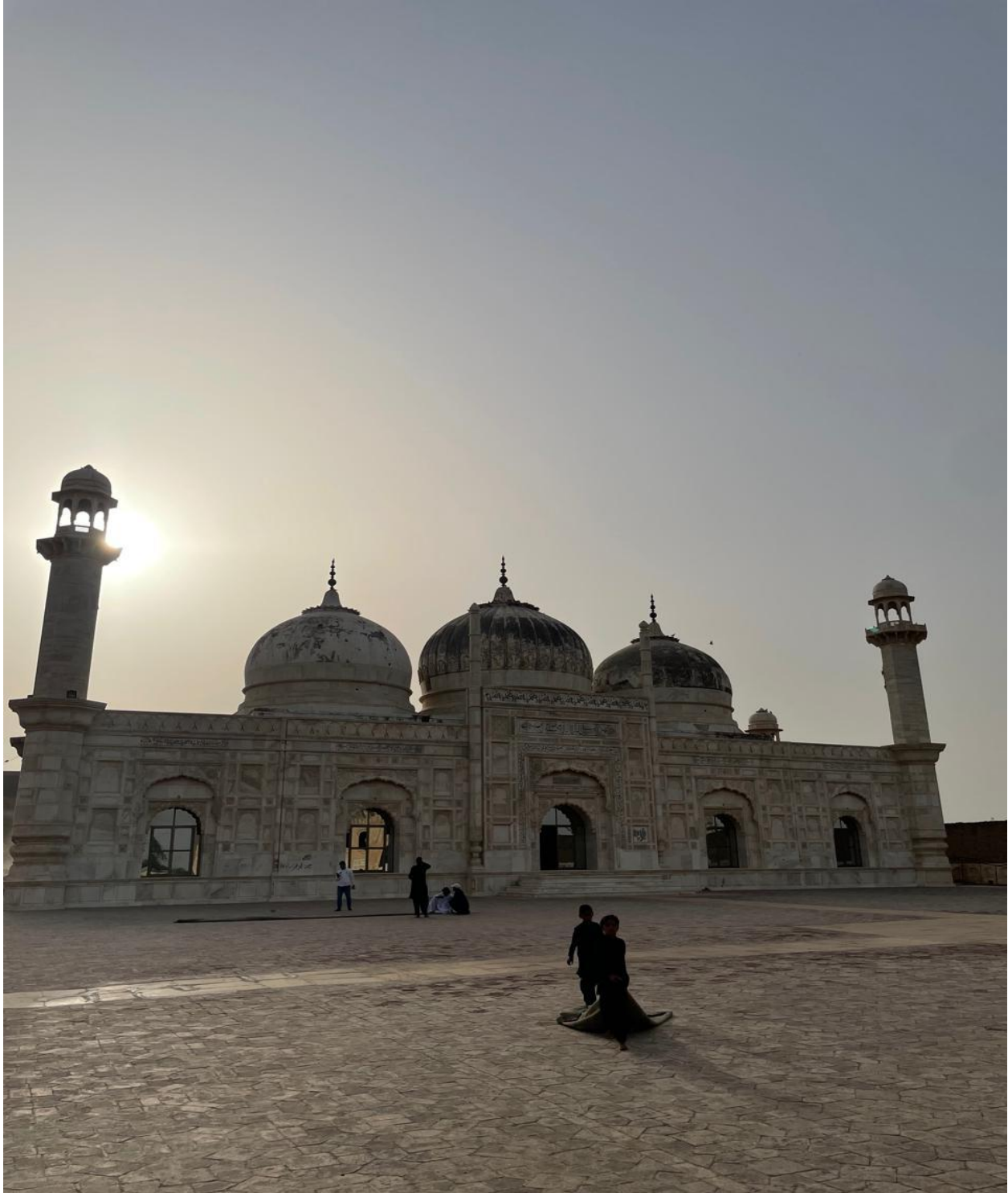
Figure 7: Abbasi Mosque Derawar
