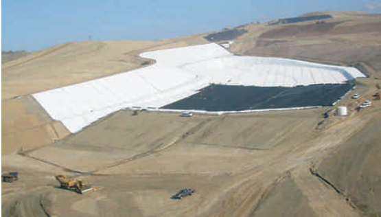
Figure 8.6: A typical canyon landfill site [6]
