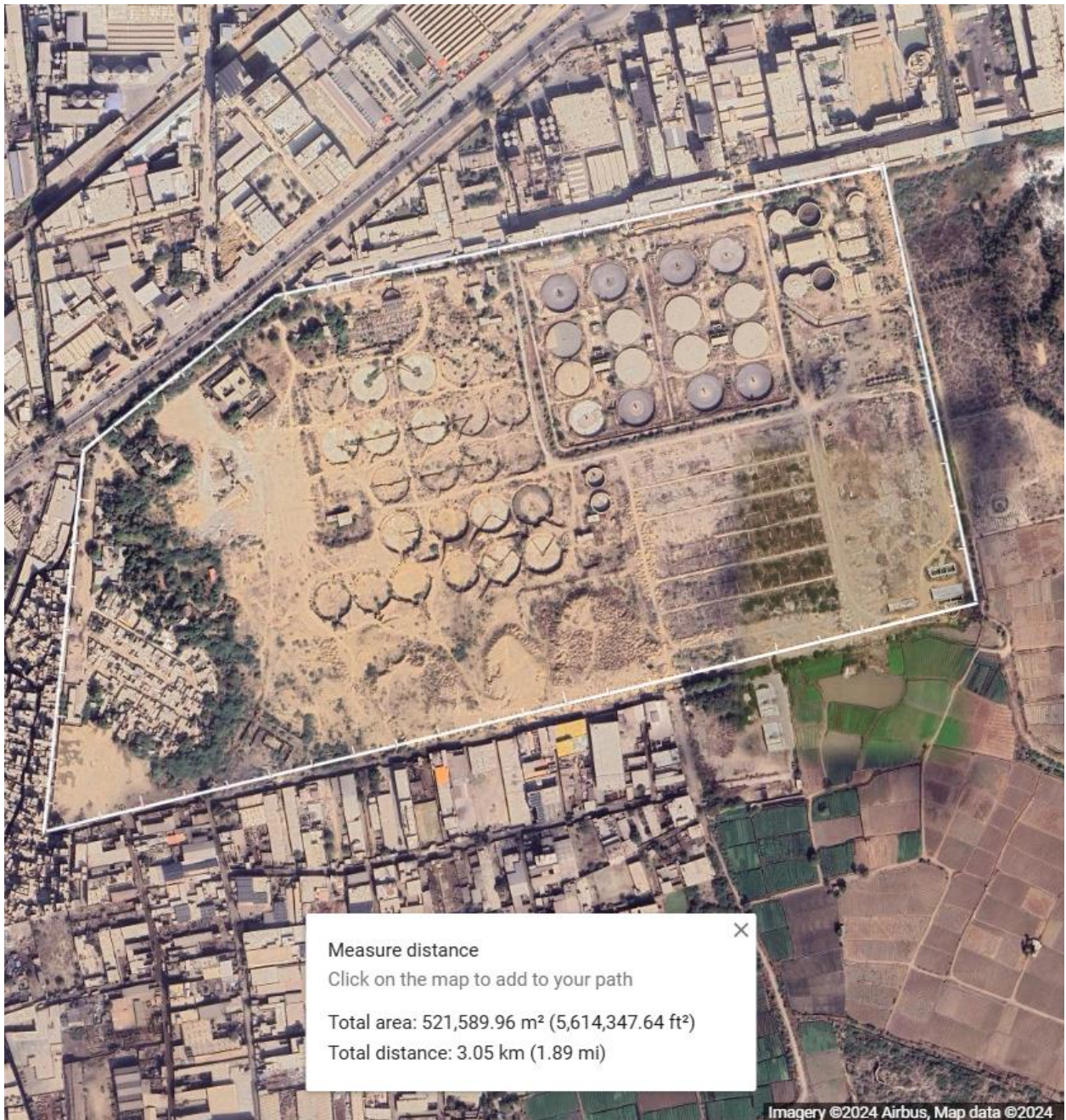
Sewerage Treatment Plant - I, Haroonabad
