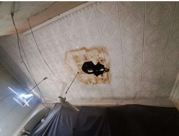
Muzaffargarh Canal Office
