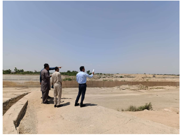
Damaged Syphon at HT X-ing
