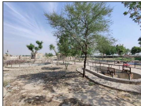
Poor condition of Disposal Station Aqilpur Road is evident from picture above.
