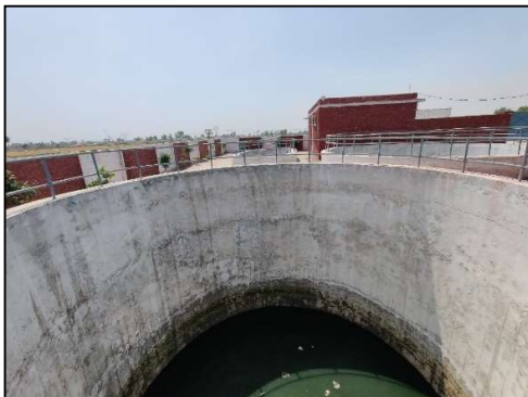
Wet Well of a newly constructed disposal station in Rajanpur city.
