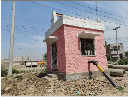
An abandoned tube-well on the Qutab Canal installed in 2007. Lack of public interest is one of the reason for abandonment.
