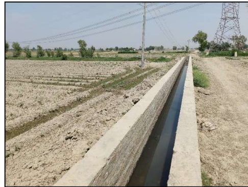
Sullage Carrier carrying wastewater for broad irrigation from the Under Construction Disposal Station Fatehpur Road.
