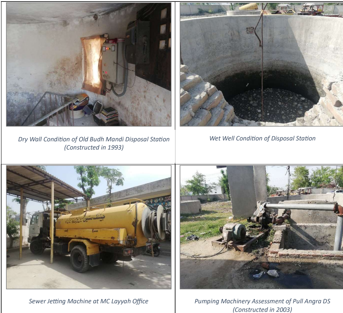
Figure 51: Sewerage System Assets condition
