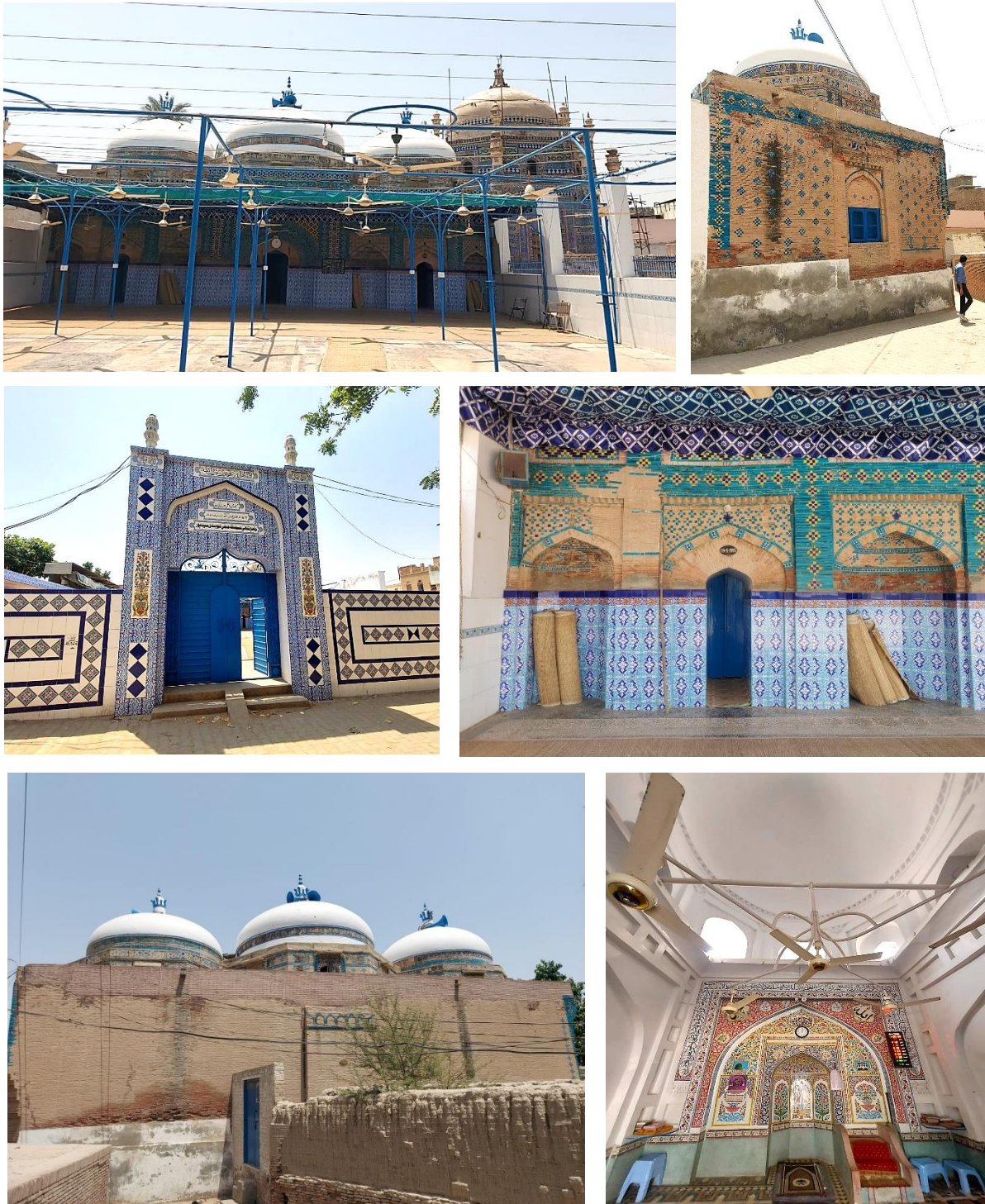
Figure 30: Existing condition of the mosque
