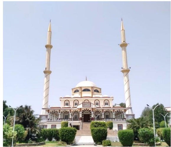
Figure 33: Existing condition of Jamia Masjid
