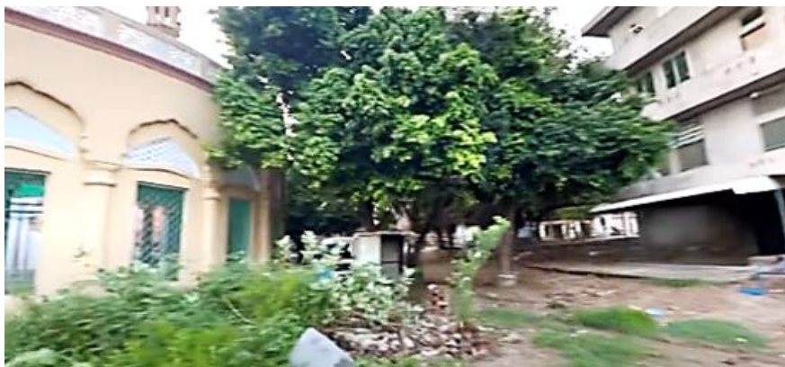
Figure 92 No plinth protection of Masjid wall
