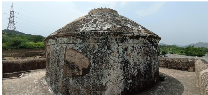
Figure 106: Crack and algae growth on plaster
