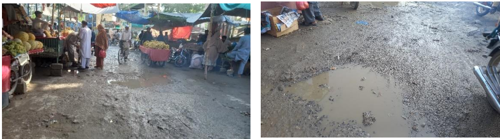
Figure 83. Condition of streets after rain
