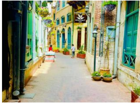
Figure 105. An example of facade uplift in a street
