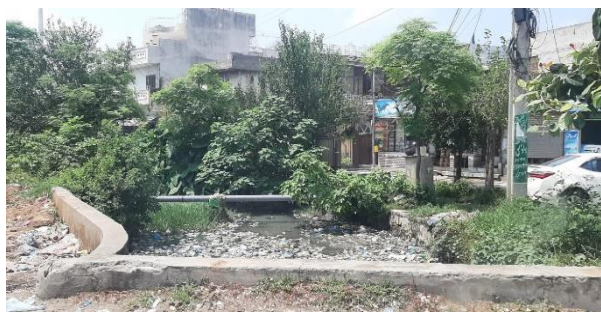
Figure 71. A large open drain outside residential colonies
