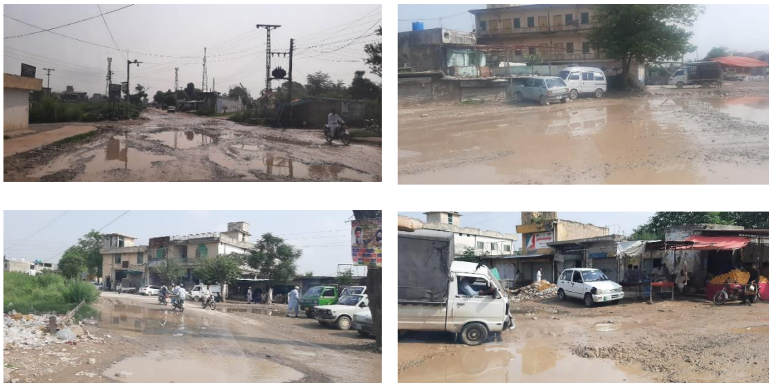
Figure 48. Poor condition of roads (especially after rainfall)
