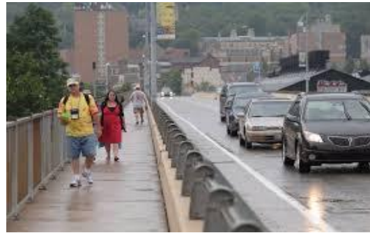
Figure 131. A Depiction of Side walkways for pedestrians
