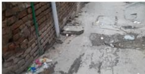
Lack of cleanliness
