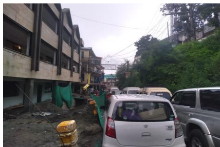
Traffic jam due to poor condition and narrow width of road
