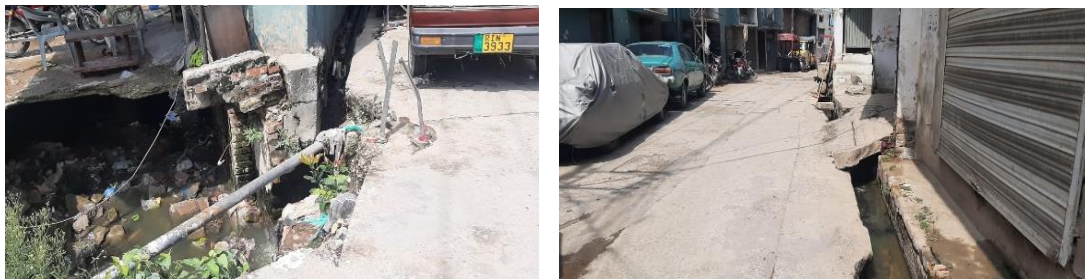
Figure 38. Open drains in residential area near Nala Lai
