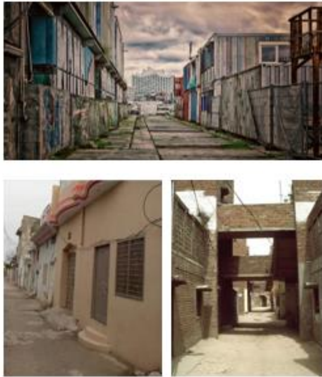
Figure 145. Images depicting façade uplift
