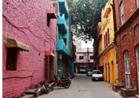
Figure 112. An example of facade uplift of a street
