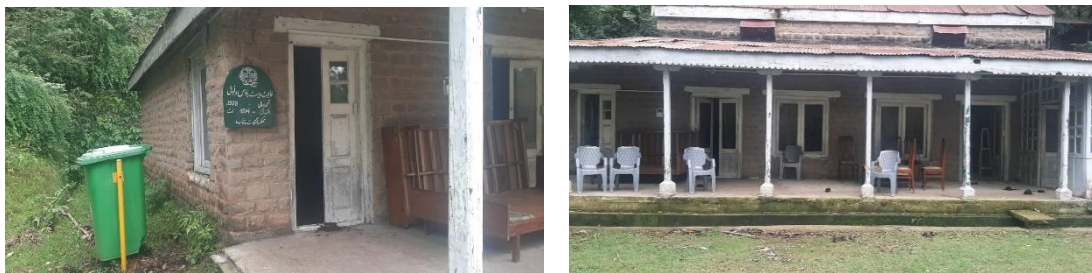
Figure 55. Forest Rest House Kotli Sattian.
