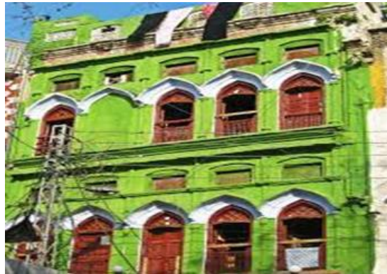
Figure 126. An example of uplifting facade
