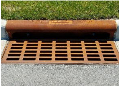
Figure 113. A depiction of how to cover open drain at sideways of streets.
