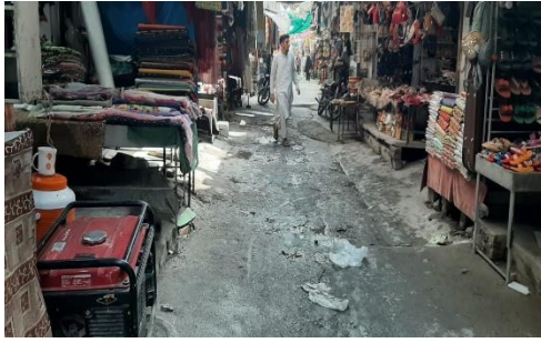
Poor condition of streets
