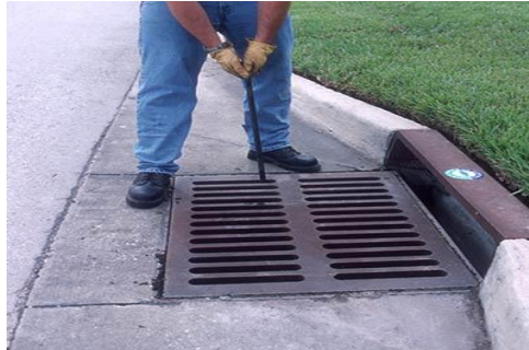
Figure 120. An example of covering open drains
