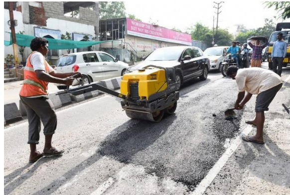
Figure 141. Repair Streets and roads
