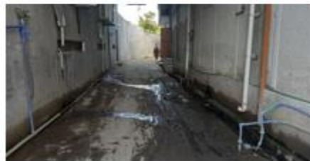
Water supply and sewer pipes together
