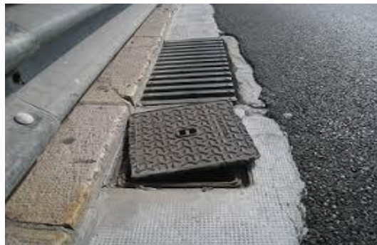
Figure 123. An example of covering open drains and manholes
