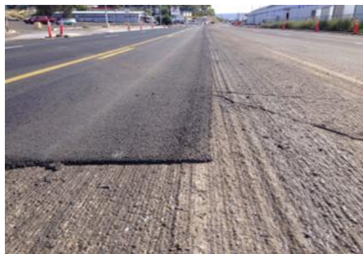
Figure 124. An example of repairing a road
