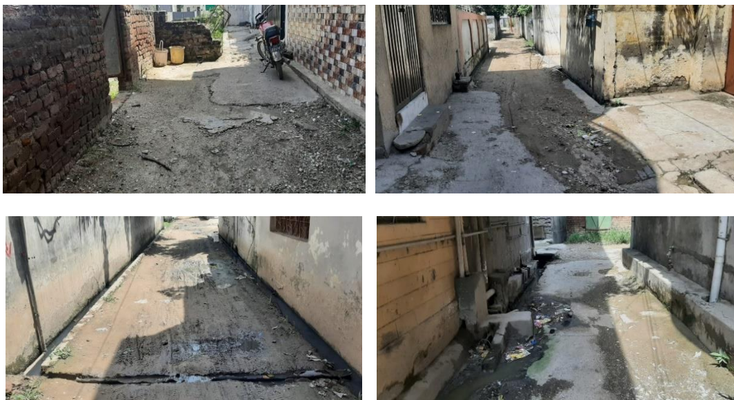
Figure 69. Poor condition of streets in several residential areas in Jhelum city
