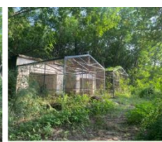
Damaged Bird Cages
