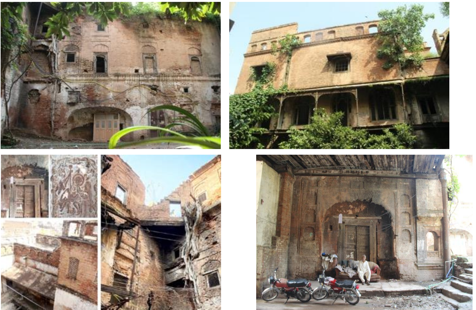
Figure 16: Pictures Shows Current Condition of Haveli
