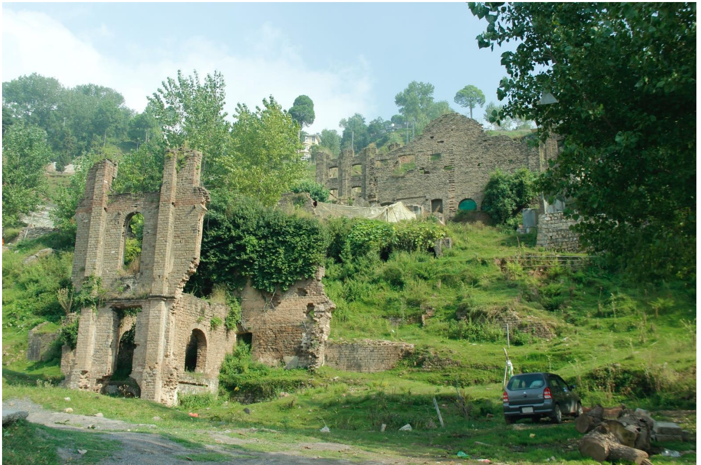
Figure 23a: Picture Shows Current Condition of Brewery
