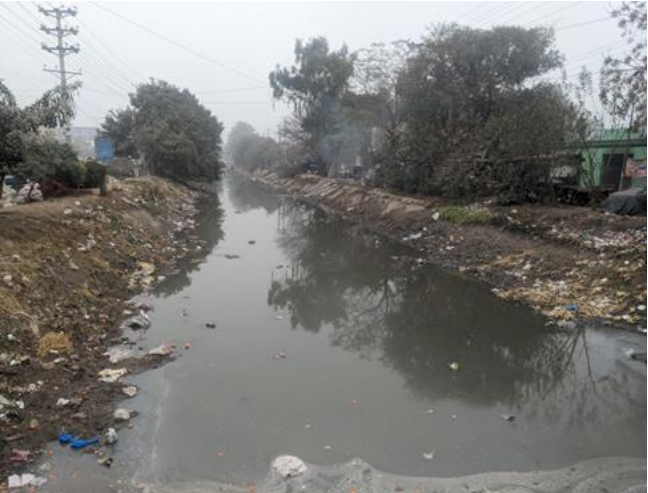
Existing condition of the proposed project site
