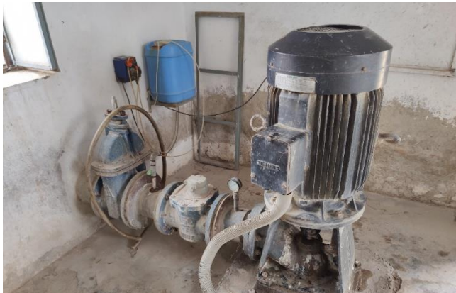
Good Condition of pumping machinery at a tube well in Pakpattan. It should be noted that all TWs in the city are equipped with proper chlorination mechanism and most have working bulk meters.
