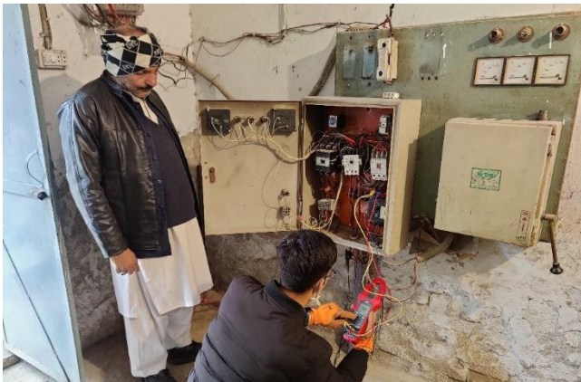
Electrical assessment being performed at a TW in Pakpattan. A power factor of 97.2% on average across 3 phases was observed. 83% Electrical Panels were found to be in Satisfactory Condition .
