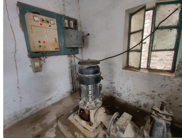
Installed in 2000, the TW in Chak 19/SP is still functional but at the verge of its design life as evident from the picture above
