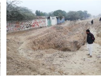
Sewer Crown Failure
