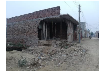
House Damage due to Sewer Crown Failure
