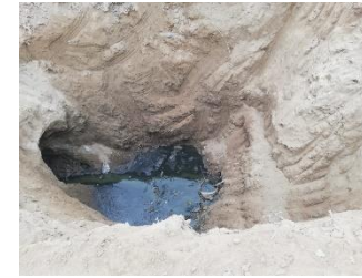
Sewer Crown Failure
