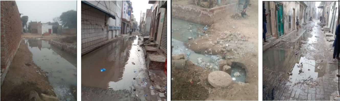
Ponding issues and poor sewage lines in Wazir colony & Aladaad Colony
