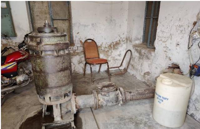
A tube well installed in 1992. The Poor Condition of the asset is evident from the over-lived pumping machinery & moisture damage on walls. 17% TWs in the city are in a similar state.
