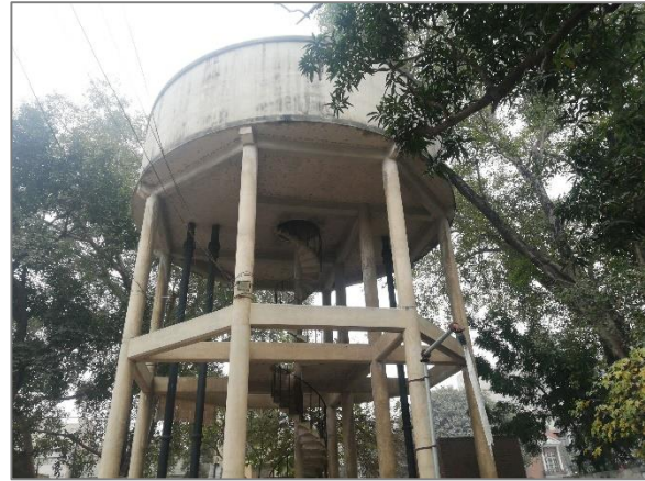
Overhead Reservoir at Old Waterworks constructed in 1935
