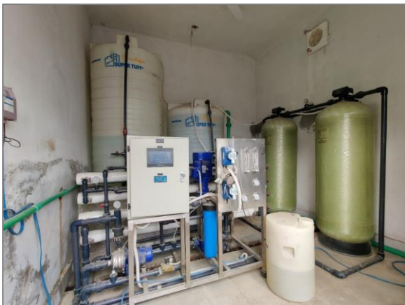
Inside view of a Rural FP Scheme. A Filtration Plant installed by Punjab Ab e Pak Authority in Chak Shafee of Pakpattan Tehsil
