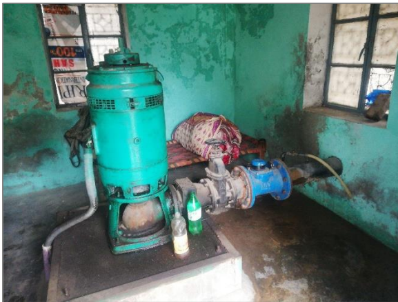
Condition of Pump House of TW#05 constructed in 2003
