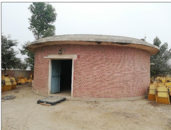
Condition of Dry Well of 1/4 L Disposal Station
