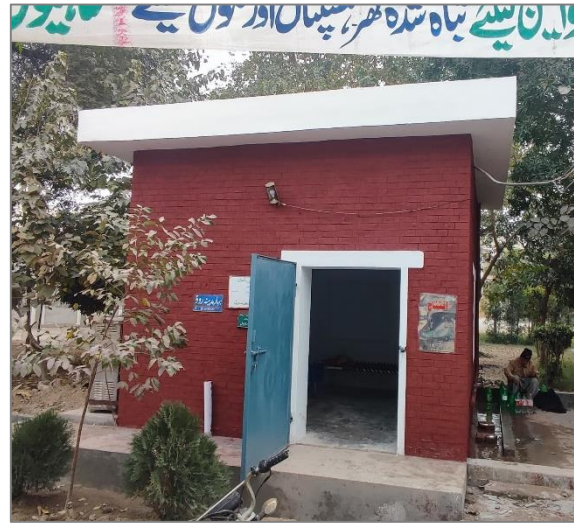
Tube well (Bahar-e-Madina Road) rehabilitated under ADB PICIIP Project
