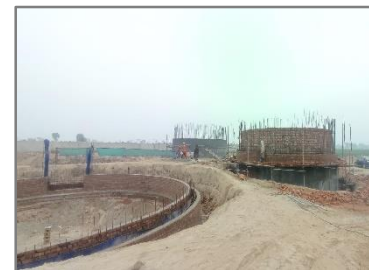
Under Construction Disposal Station (North)
