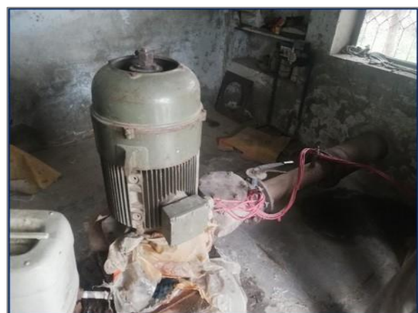
WS Scheme Dharmay Wala – Depalpur Rural Scheme in Brackish Zone/ House Connections: 550 Nos. Poor Condition of TW Pump House Observed. Rehabilitation of Civil Structure of TW Pump House and Electromechanical Machinery required
