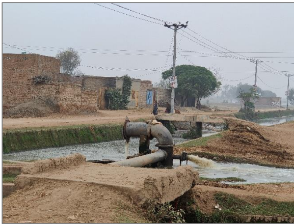
Direct disposal of wastewater in irrigation channel in MC Pakpattan.
