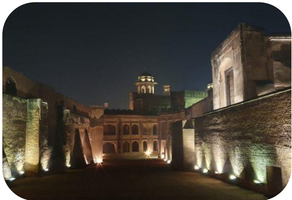
Night illumination to enhance safety and security and promote heritage sites.
