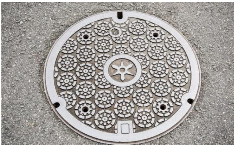
Figure 88: Covered Drain enhancing quality of streets and roads
