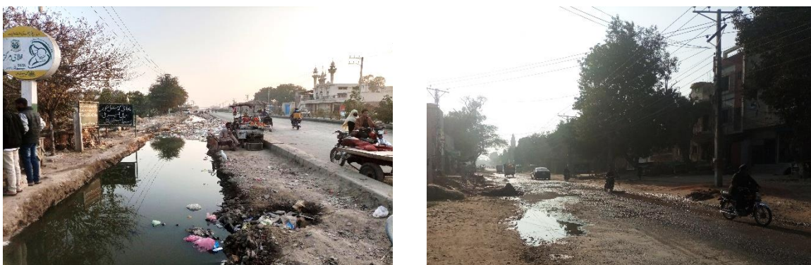
Figure 45: Condition of Sanitation at Inayat Elahi Katchi Abadi & Harappa Road, Sahiwal.
