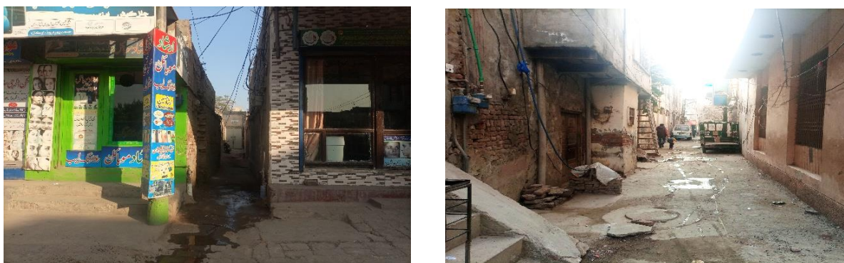
Figure 49: Condition of Streets in Ahmedabad Colony and Kumhar Muhallah, Okara.
