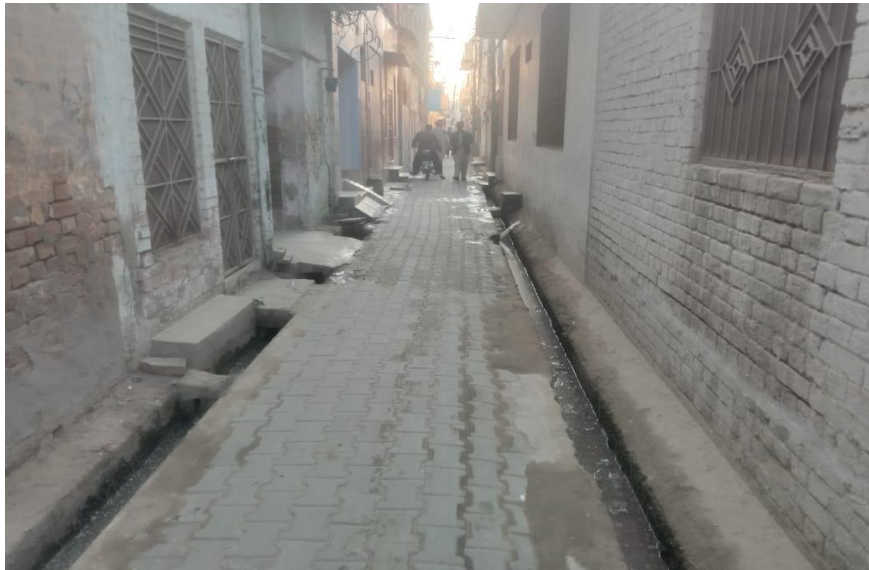
Figure 27: Situation of Street Drainage Network in Pakpattan.
