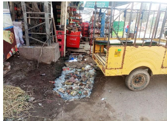
Figure 51: Open drains with clogging issue due to solid waste in residential and commercial areas of Okara
