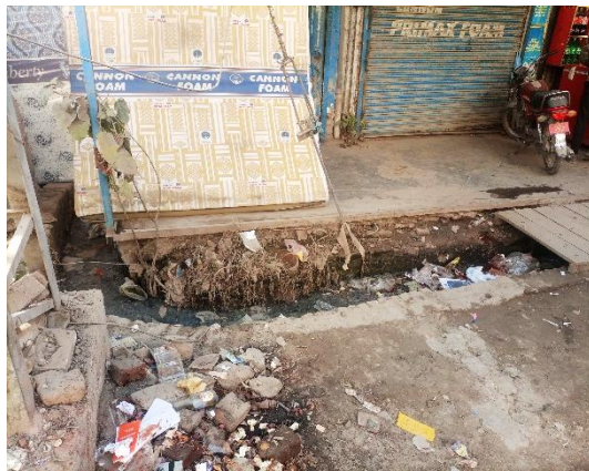
Figure 51: Open drains with clogging issue due to solid waste in residential and commercial areas of Okara
