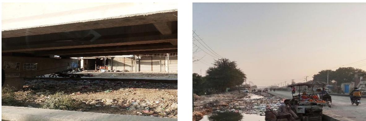
Figure 48: Open Dumping of Solid Waste along roads and under the flyovers.
