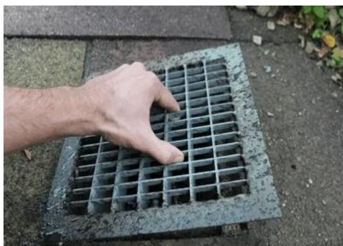
Figure 82: A depiction of how to cover open drain at sideways of streets
