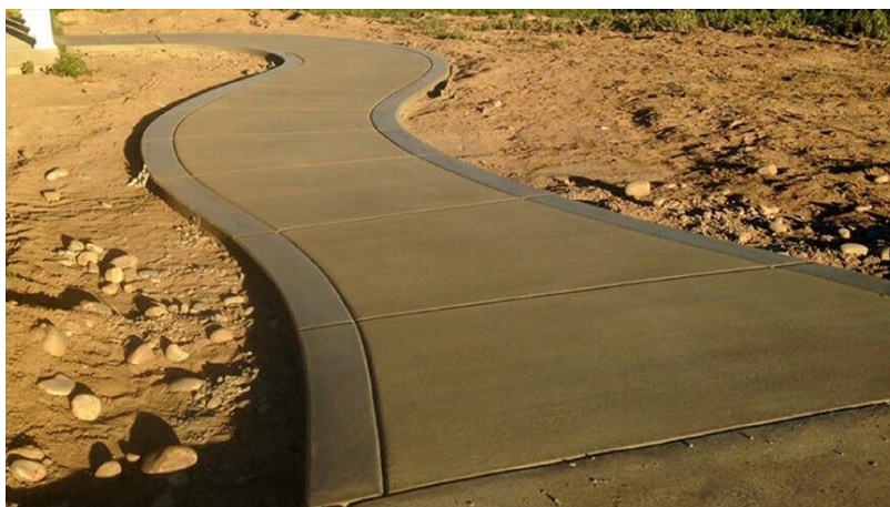
Figure 108: Paving of Streets and Road Surface
