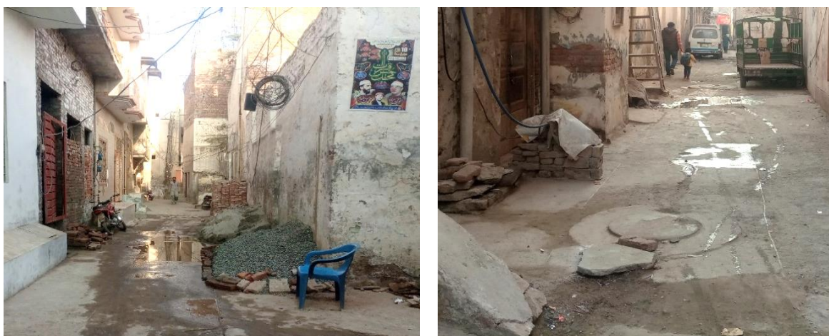
Figure 100: Depiction of Poor Street Infrastructure at Kumhar Muhallah, Okara
