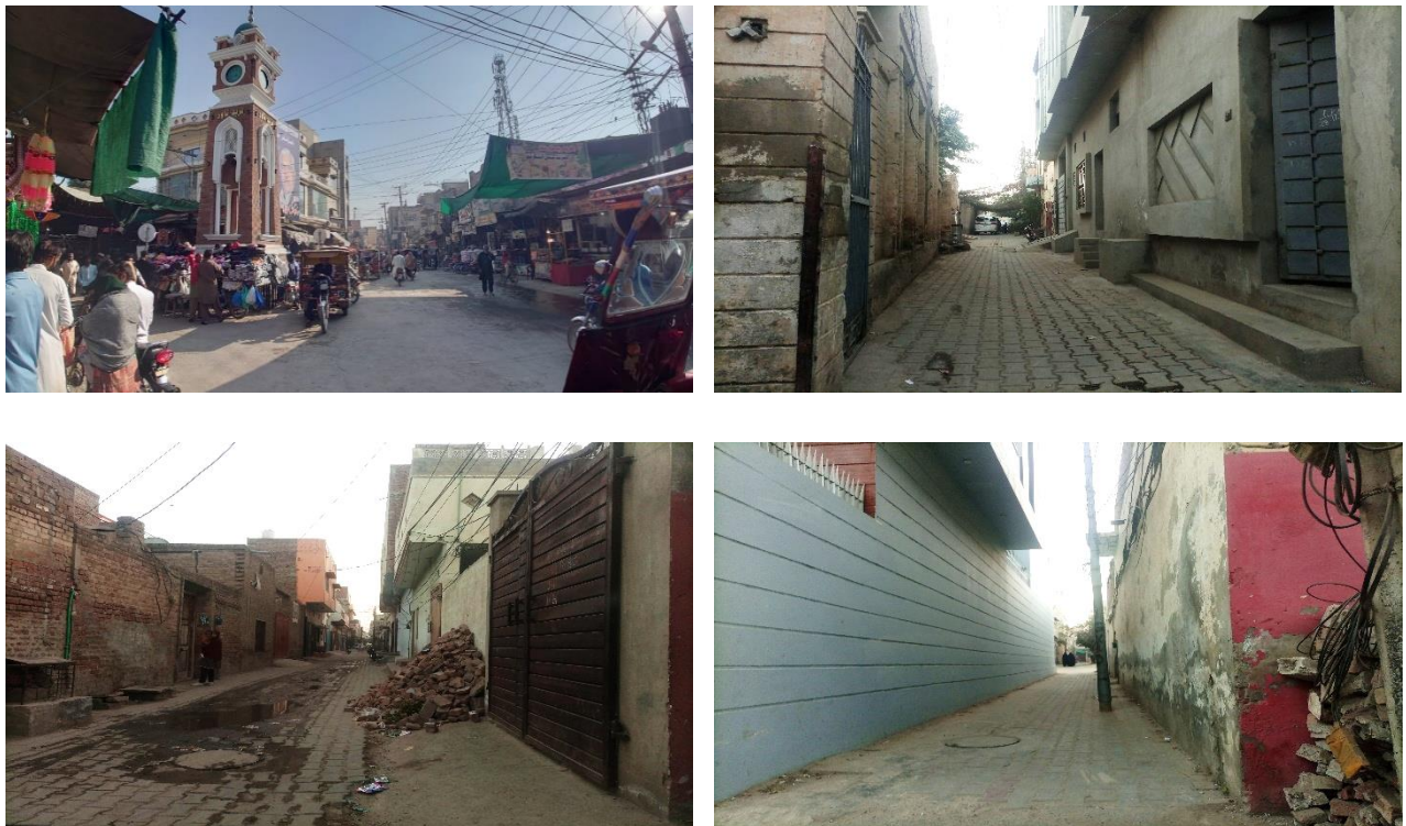
Figure 90: Existing condition of Urban Area around Darbar Hazrat Baba Farid-ud-din Ganj Shakar, Pakpattan
