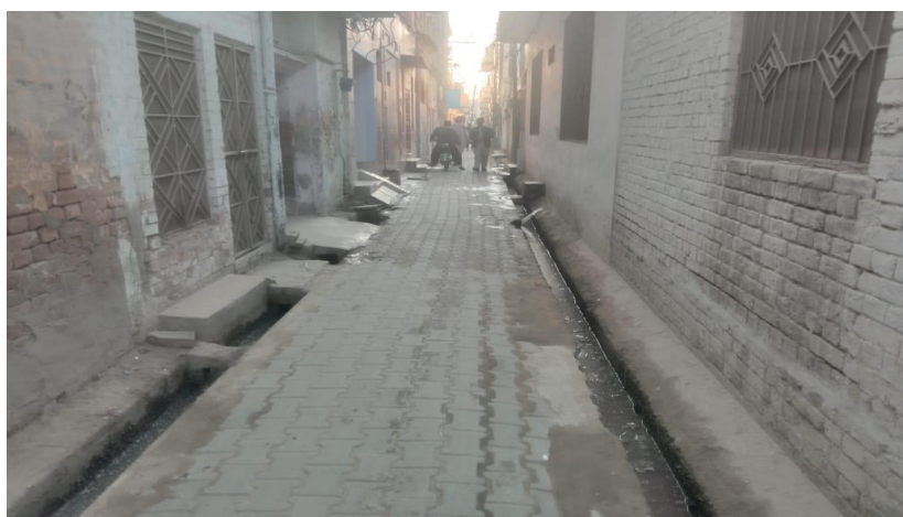
Figure 103: Open Drainage Links in street
