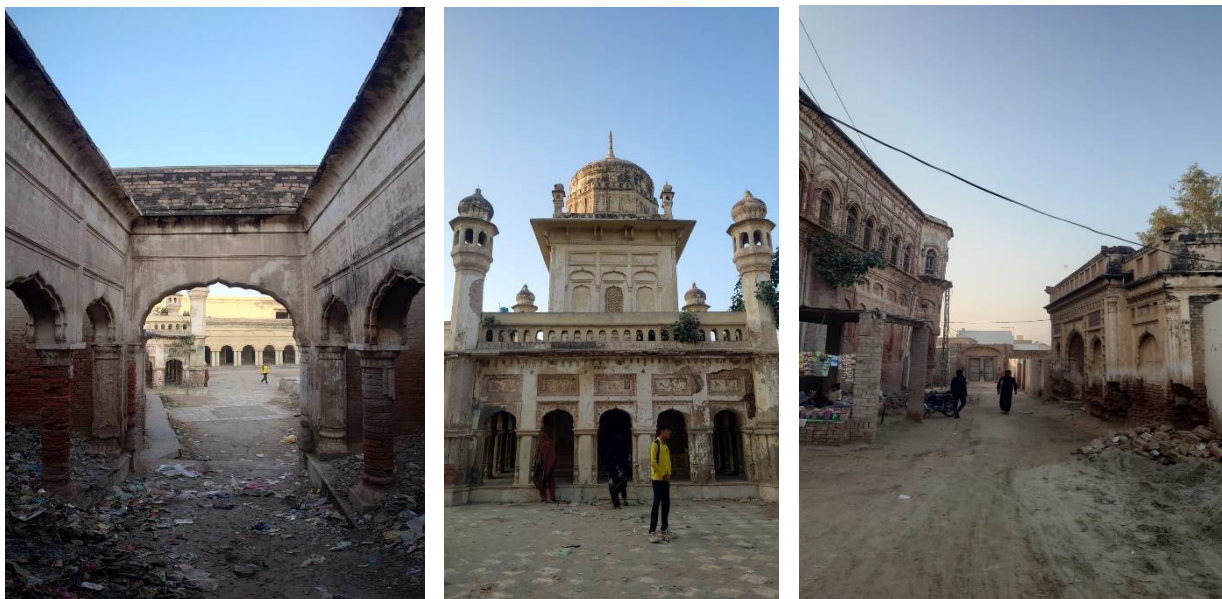
Figure 28: (left) Dilapidated/vandalized structure inside complex (mid) gurdwara Front elevation (right) Entrance route.
