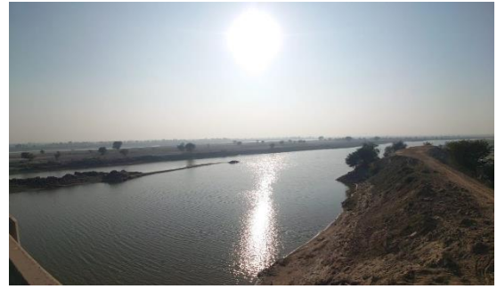
Figure 44: River Sutlej view from bridge.
