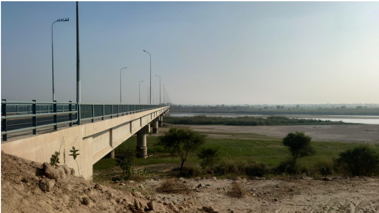
Figure 16: River Ravi bridge Sheraza Pattan
