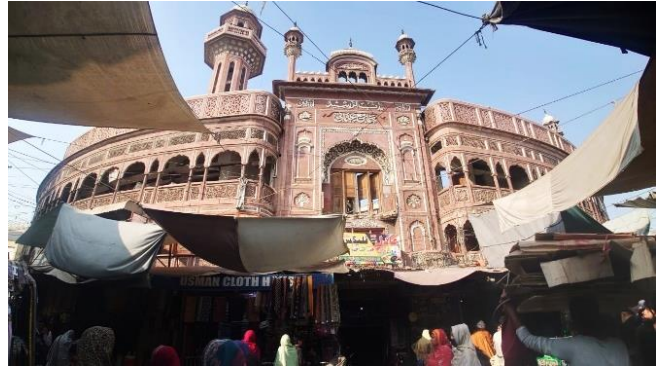
Figure 23: Gol Masjid Exterior
