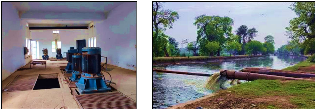
Figure 22: Field Survey and Assessment
