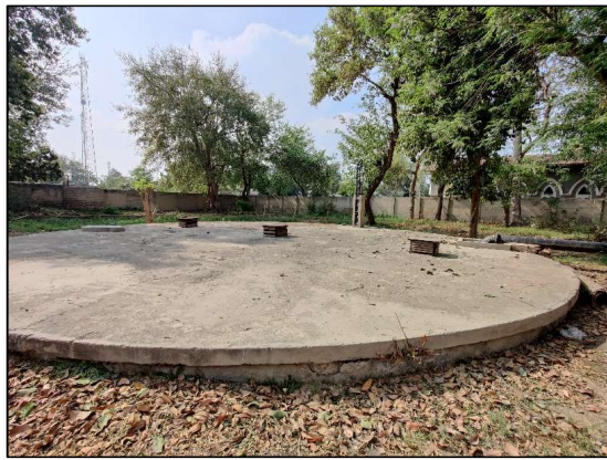
Ground Storage Tanks, Vehari
