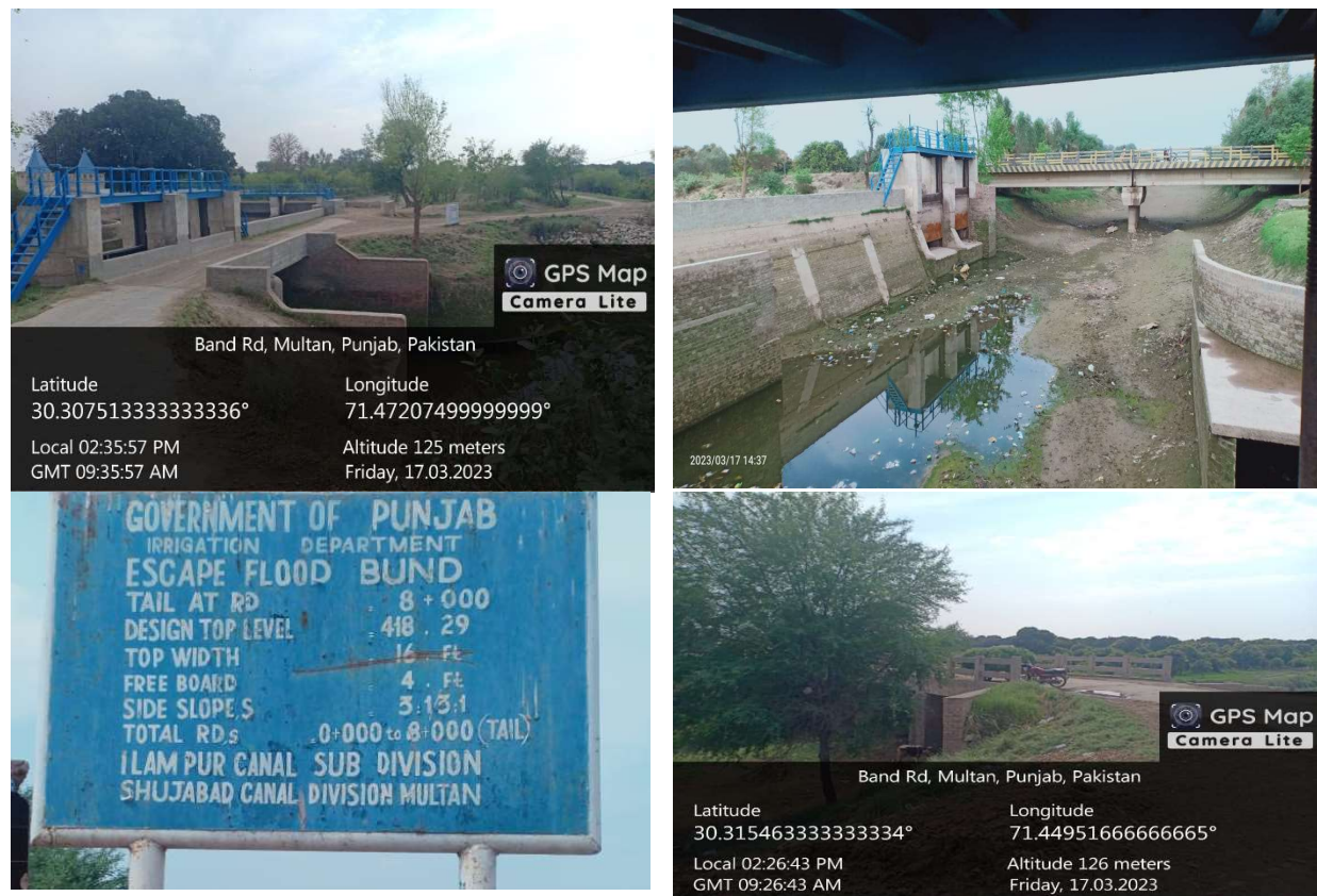
Figure 8: Flood Escape Bund at Nawabpur Rest Area of Shujabad canal circle.
