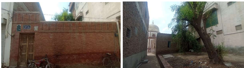
Figure 44: Access to Mai Meharbaan Tomb and its entryway
