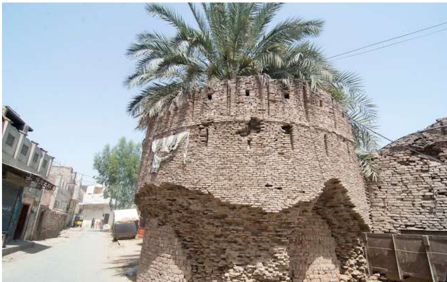
Figure 79: One of twelve bastions in the exterior fortification wall
