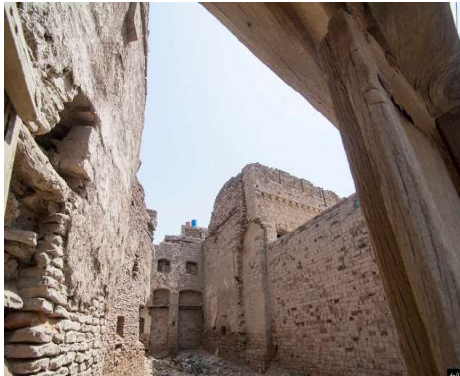
Figure 81: Internal wall now surrounded by newly built houses
