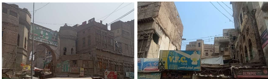
Figure 38: Built fabric surrounding Bohar Gate
