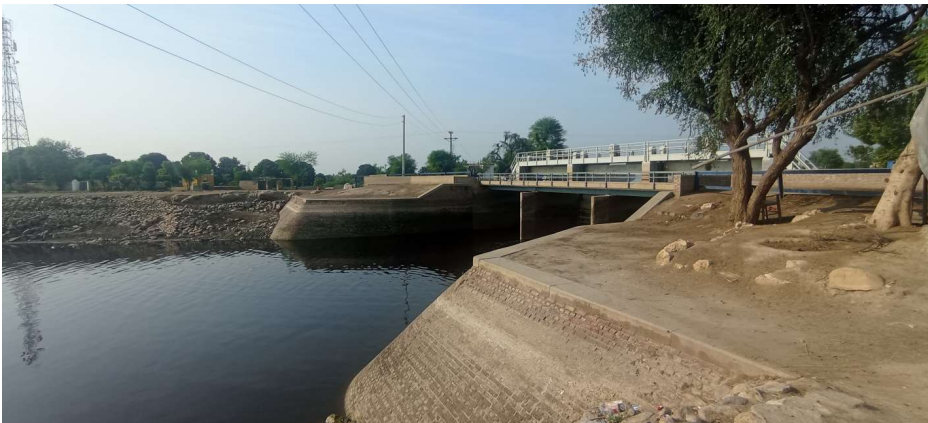
Figure 23: Sher Garh Headworks
