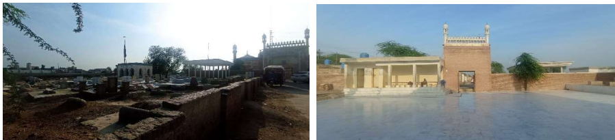
Figure 88: Existing condition of Shahi Mosque
