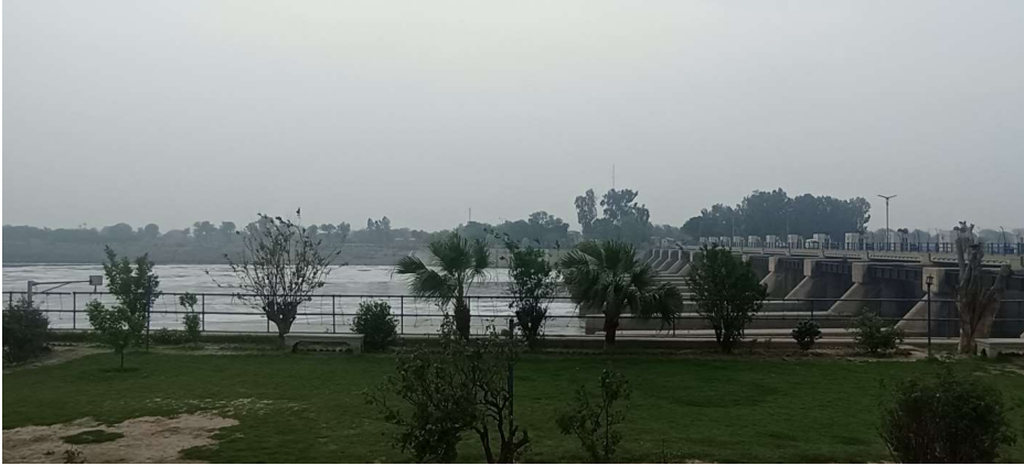
Figure 22: Headworks view from the park
