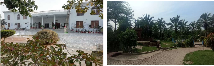
Figure 97: Existing condition of Faisal Masood Jhandir library
