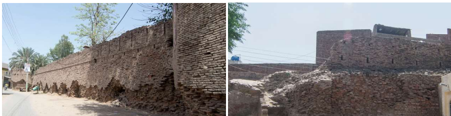
Figure 80: Existing wall and remains of Tulamba Fort
