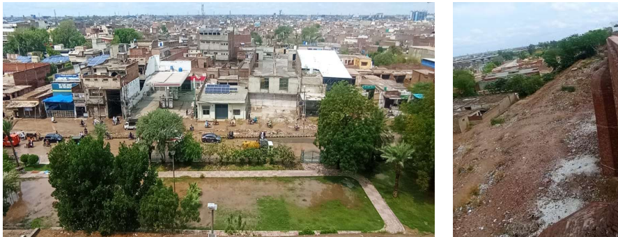
Figure 31: Existing condition of identified site for food street
