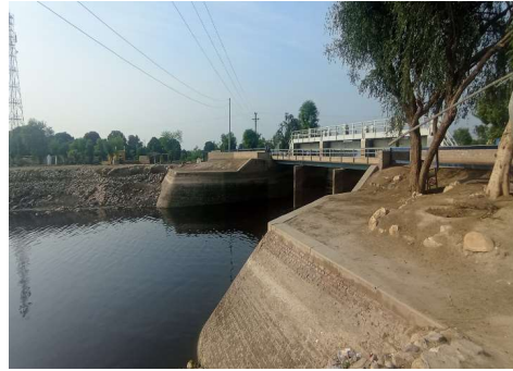
Figure 92: Headwork shergarh mailsi
