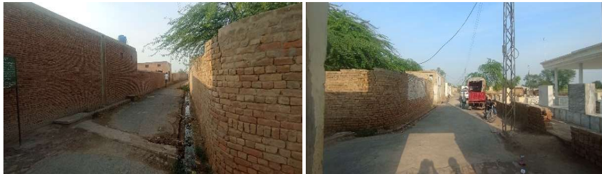
Figure 90: Adjacent Road and parking facilities
