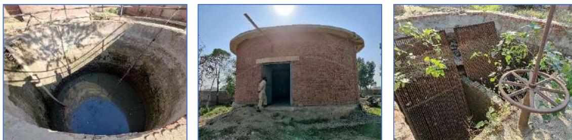
Figure 56 Condition of Civil Components of Sewerage Infrastructure
