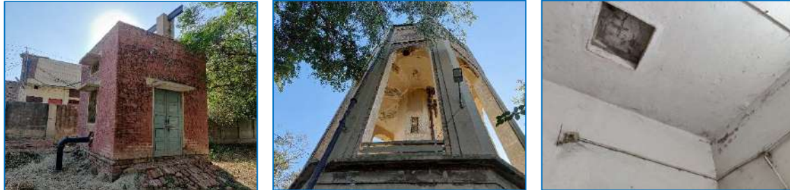
Figure 48 Condition of Civil Components of Water Supply Assets
