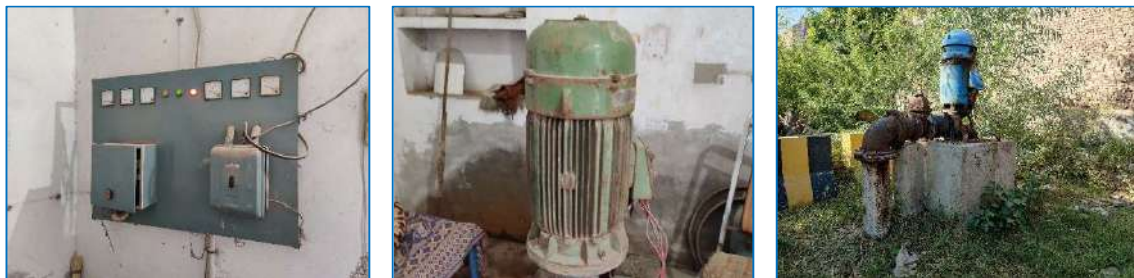
Figure 49 Condition of Electro-Mechanical Components of Water Supply Assets
