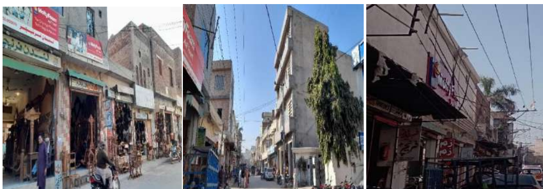
Figure 81: Building facade and Encroachment on Road
