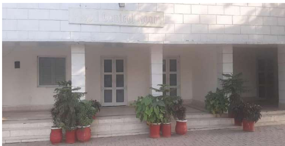
Figure 35. Flood Control Room at Chenab River near Trimoo Barrage
