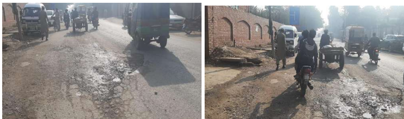
Figure 31. Existing condition of a major road, in Jhang
