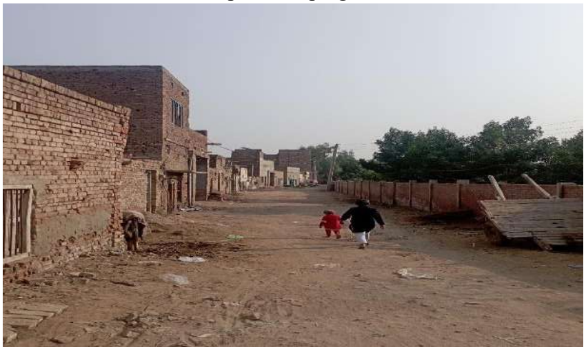
Condition of Houses and Street
