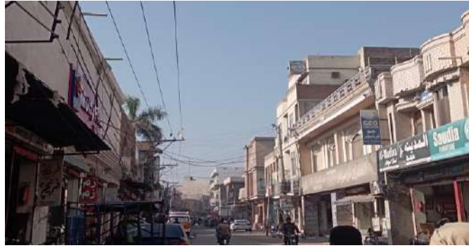
Encroachment on Roads
