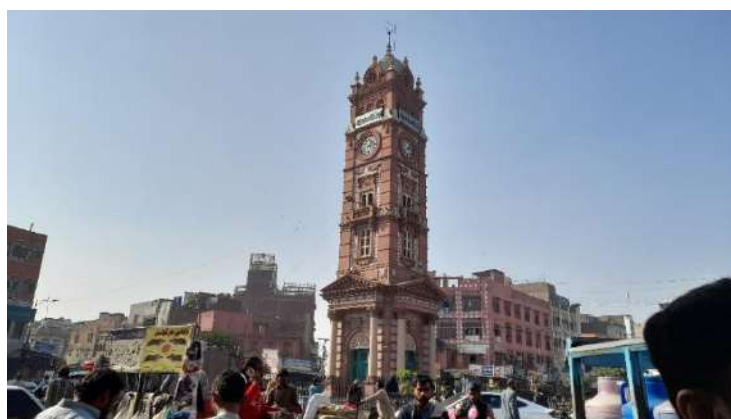
Figure 8. Faisalabad Clock Tower
