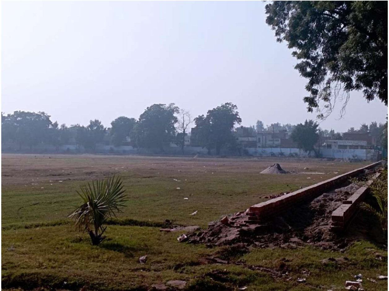
Figure 48: Lack of maintenance at the Mai Heer Stadium, Jhang
