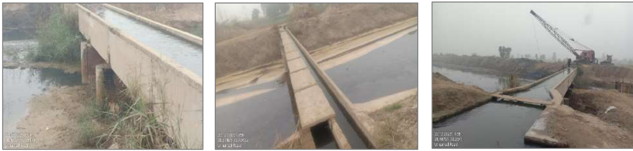
Figure 7: Condition of Aqueducts in Faisalabad
