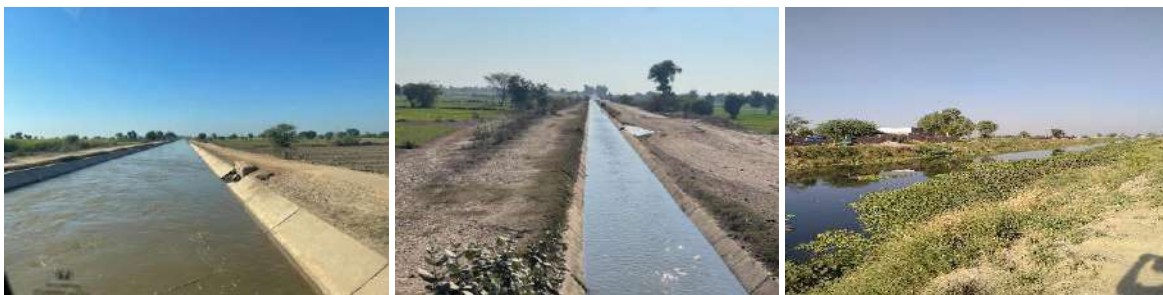
Figure 30. Existing Condition along Water Channels
