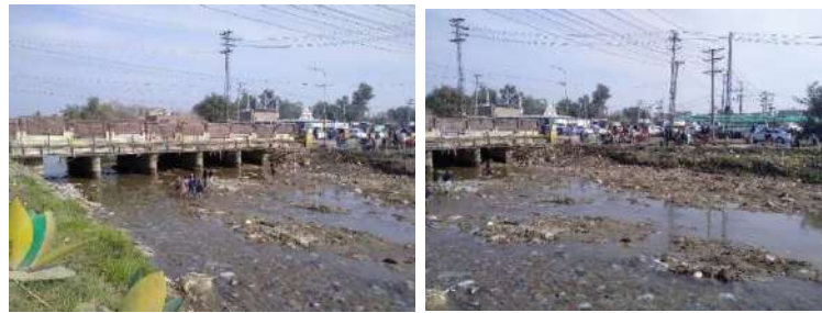
Figure 32: Current situation of Sargodha Canal
