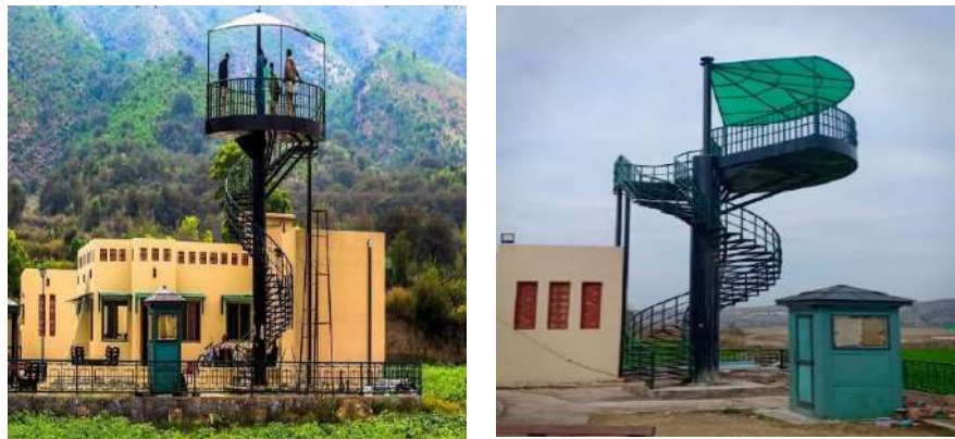
Figure 31: Examples of Bird Watching Tower of Soon Valley Project
