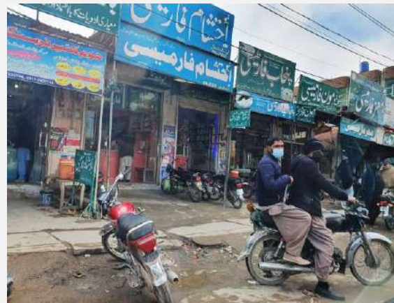
Poor drainage and footpaths
