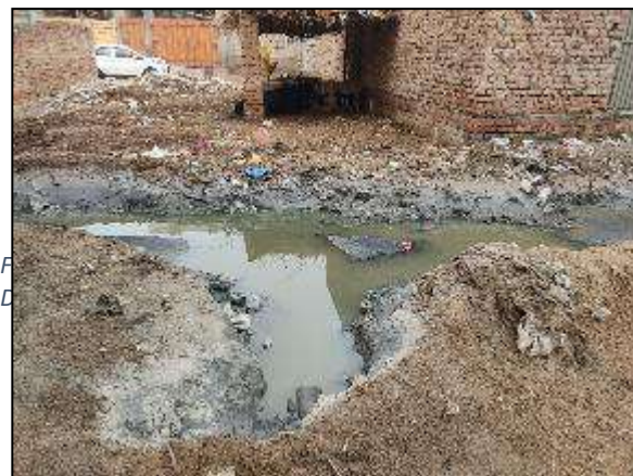
Figure 20: Overflowing waste water from Ghani Park Disposal
