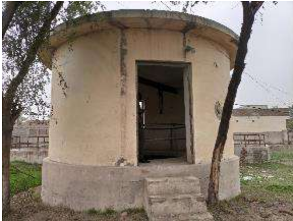
Figure 58: Disposal Station in MC Bhakkar
