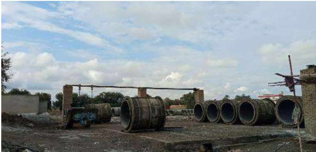
Figure 67: RCC Sewer pipes being casted for PHED Sewerage Scheme
