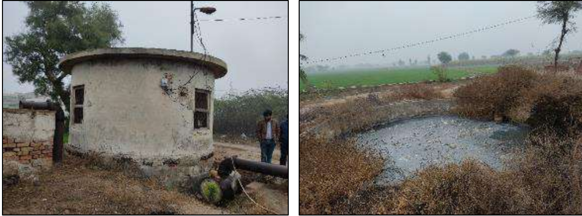
Figure 35: Disposal Station Satellite Town Khushab
