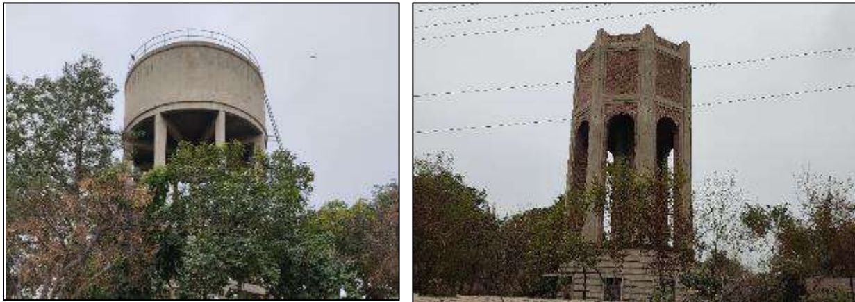
Figure 42: Overhead Reservoirs across Mianwali City
