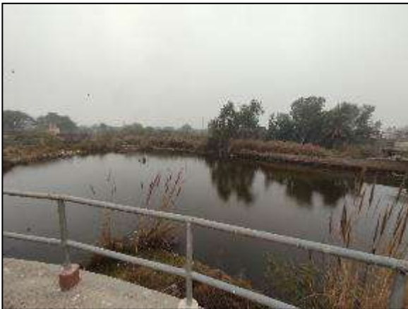
Figure 27: Water Ponding beside Rehmatwala GST
