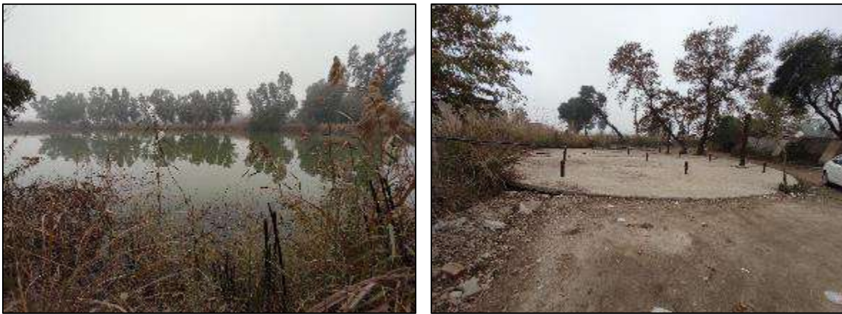
Figure 25: Water Pond and GST at Water Works (Scheme No 2) in Khushab
