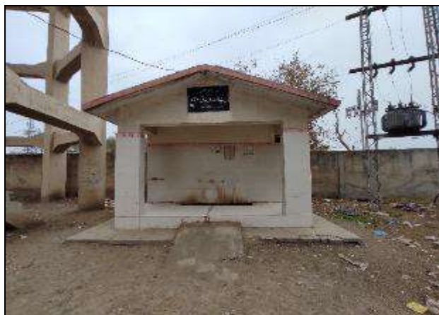
Figure 43: Filtration Plant in Mianwali City
