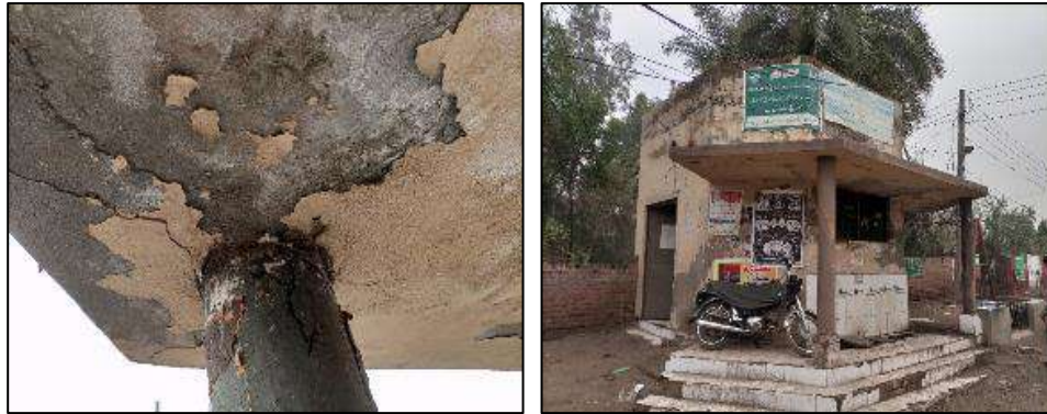
Figure 16: Filtration Plant at Katcheri Road, Sargodha
