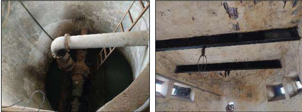
Figure 21: Well and Roof Girders of Jinnah Colony Main Disposal
