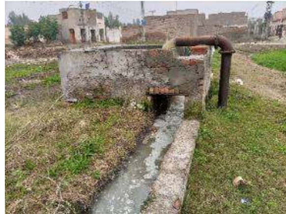
Figure 59: Waste Water being carried to fields
