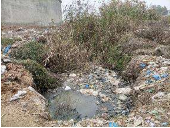
Figure 62: Water Ponding in Bhakkar City
