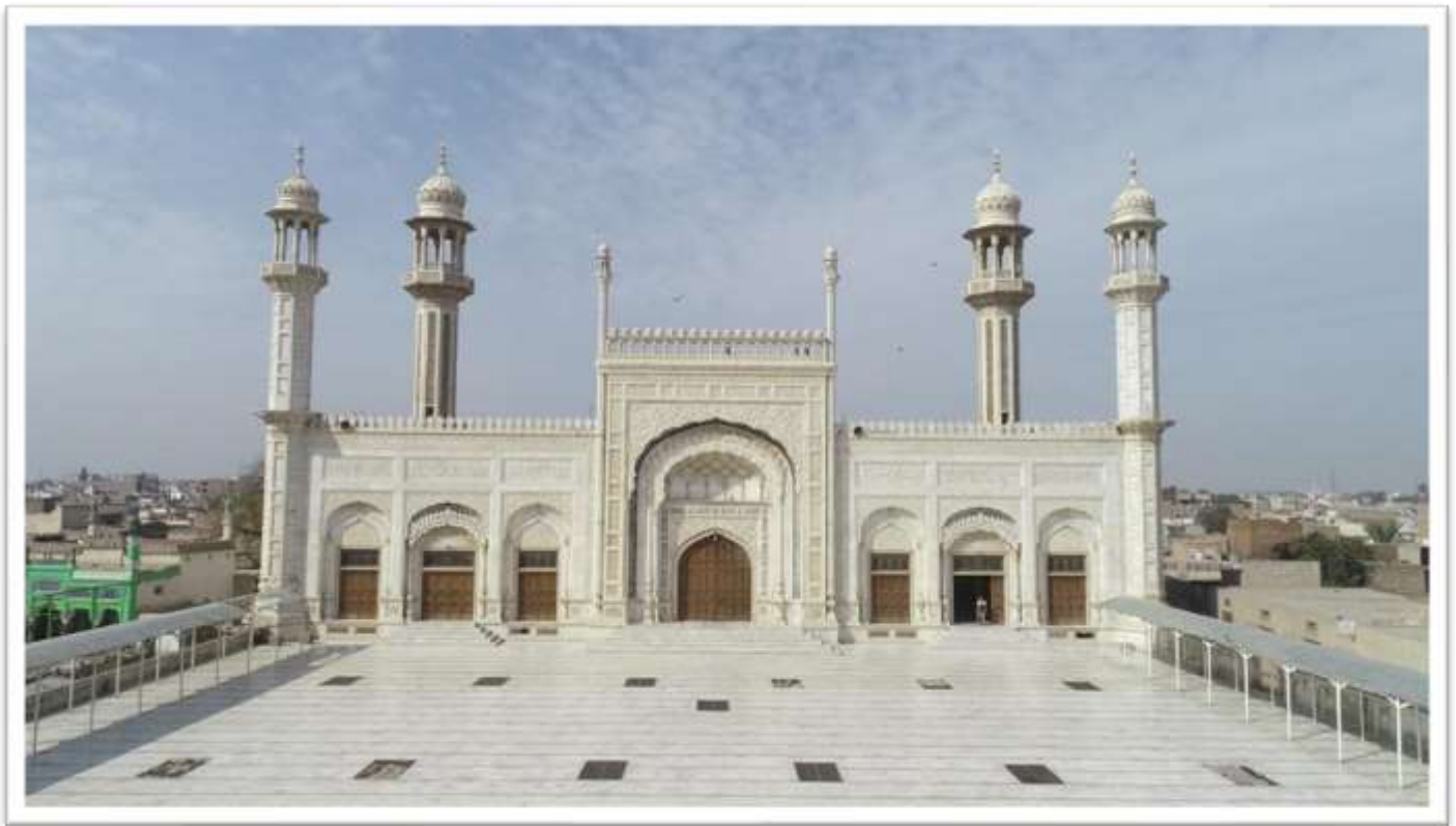
Figure 81 Al-Sadiq Mosque, State Period, Bahawalpur
