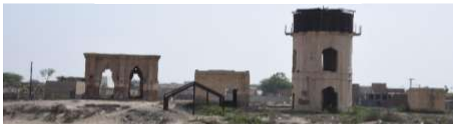
Figure 75 The Structures at the Railway Station
