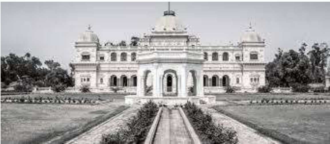
Figure 57 Different views of Sadiq Garh Palace
