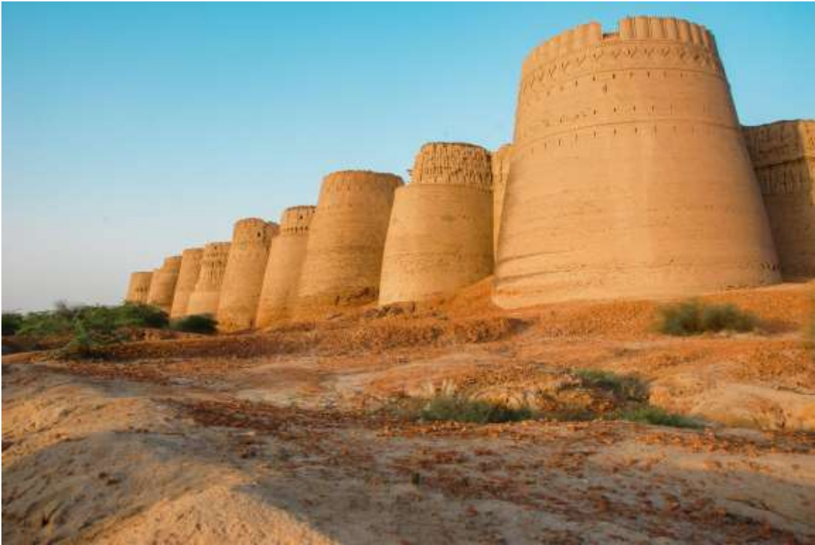
Figure 17 Side View of Derawar fort
