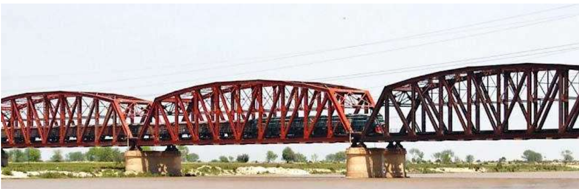
Figure 62 Colonial Period Railway Bridge, Bahawalpur
