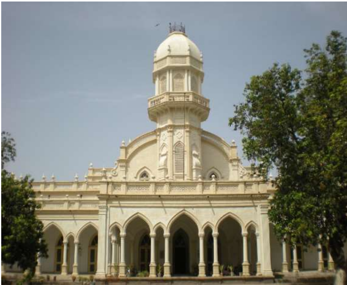
Figure 67 Façade of Central Library, State Period, Bahawalpur
