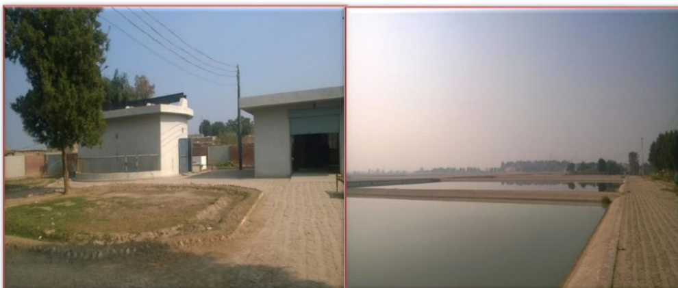
Figure 56: WSP WWTP at Moh Mubarak in RYK City
