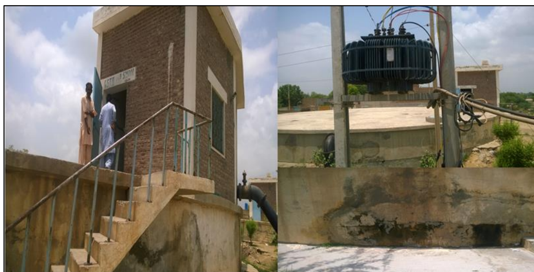
Figure 38: Ground Storage Tank in Bahawalpur City
