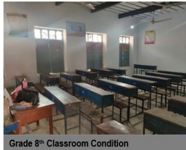
Grade 8 th Classroom Condition
