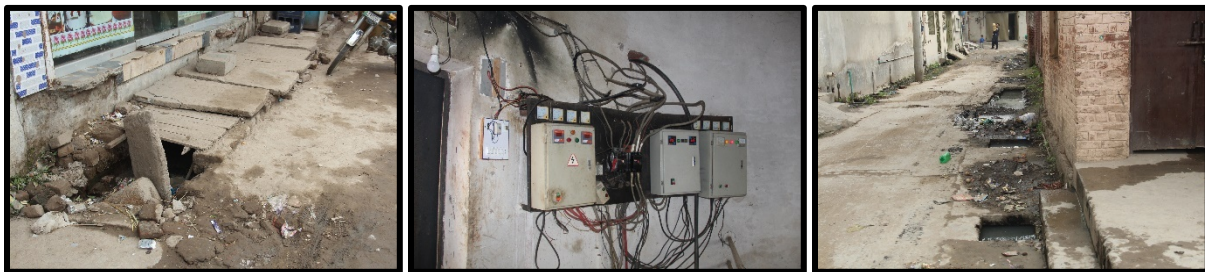
Figure 20: Condition assessment of existing sewerage system
