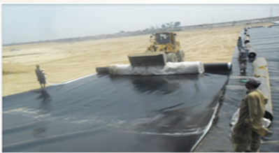
Layering of Geo Membrane
