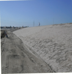
Preparation of Stabilized Embankments
