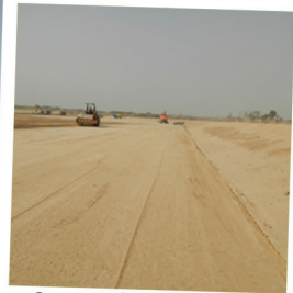
Compaction of the Final Clay Layer
