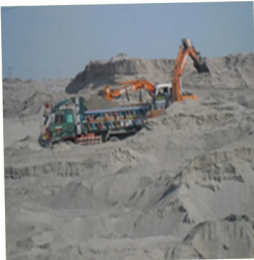
Excavation in Cell-1
