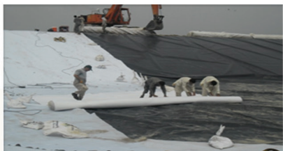
Layering of Geotextile
