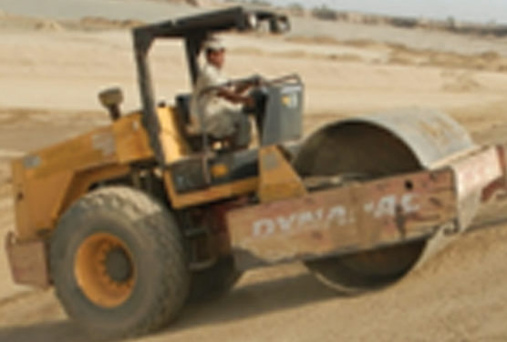
Compaction of Side Slopes of Cells
