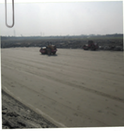
Compaction of Local Soil
