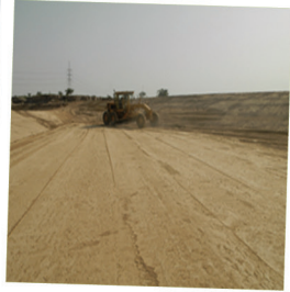
Grading of the Clay Layer
