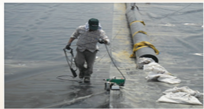
Layering of Geo Membrane
