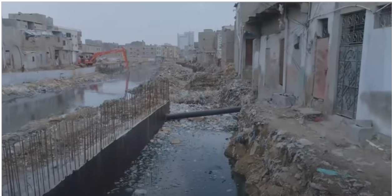
Figure 59. Blockage of Drains and Encroachments in Karachi in One Frame 99
